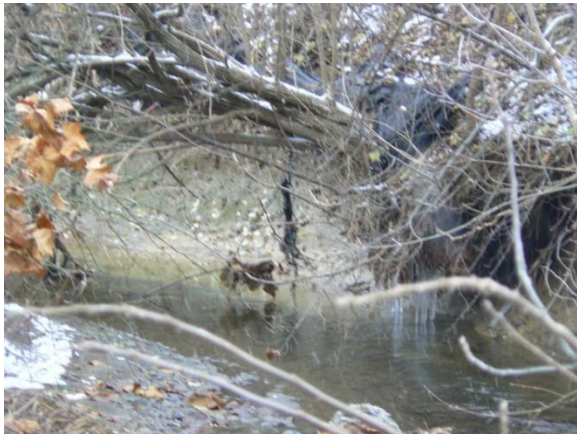
Streambank erosion along Bennetts Run, parallel to Fairfield Road - Site FPR-5. (351: 11/20/2008 – 1:30 pm)
