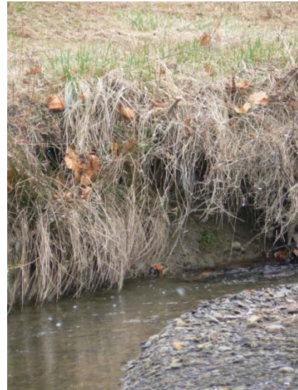
Streambank erosion along Bennetts Run, parallel to Fairfield Road - Site FPR-5. (354: 11/20/2008 – 1:34 pm)
