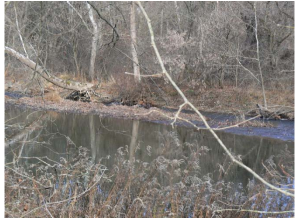
Streambank Erosion, and failing riparian zone, at Site FPR-8. (322: 11/19/2008 – 1:07 pm)
