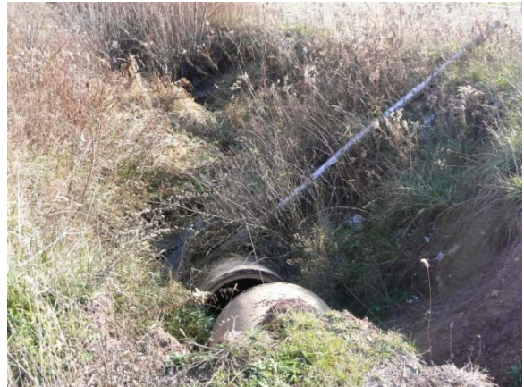
Channelized stream drainage across agricultural field, at Site FPR-6. Bank erosion is apparent. (326: 11/19/2008 – 1:33 pm)
