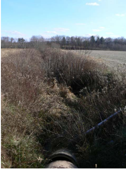
Channelized stream drainage across agricultural field, at Site FPR-6. (325: 11/19/2008 – 1:32 pm)
