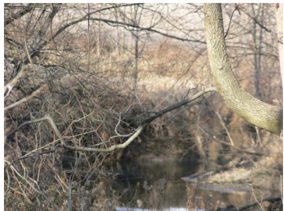
Streambank erosion along Wolf Run, at Site FPR-6. (328: 11/19/2008 – 1:37 pm)
