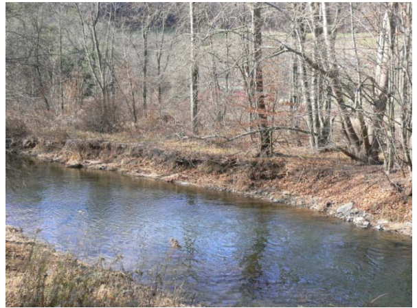
Streambank Erosion, and failing riparian zone, at Site FPR-7. (310: 11/19/2008 – 12:15 pm)
