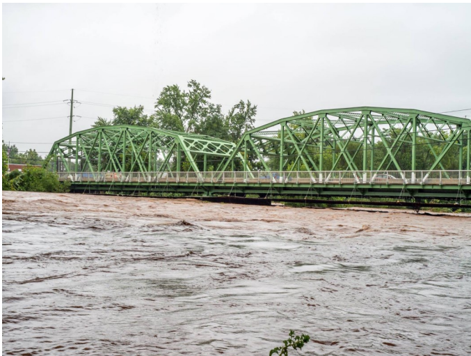
Green Bridge, Montoursville
