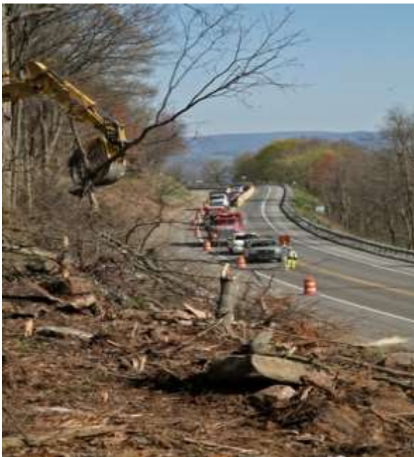
US 15 (Montgomery Pike) Safety Barrier (Photos Courtesy of PennDOT)
