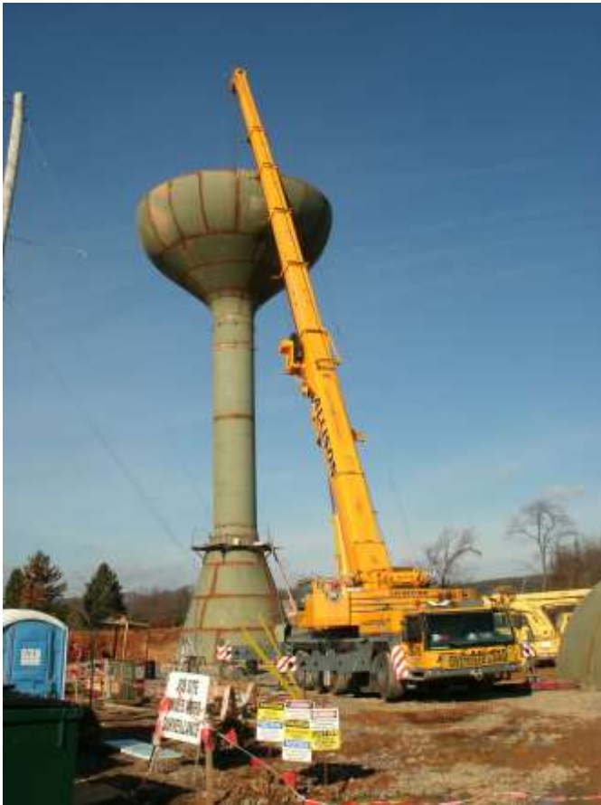
Grey Fox Plaza 200,000 gallon elevated water storage tank installed during summer 2011
