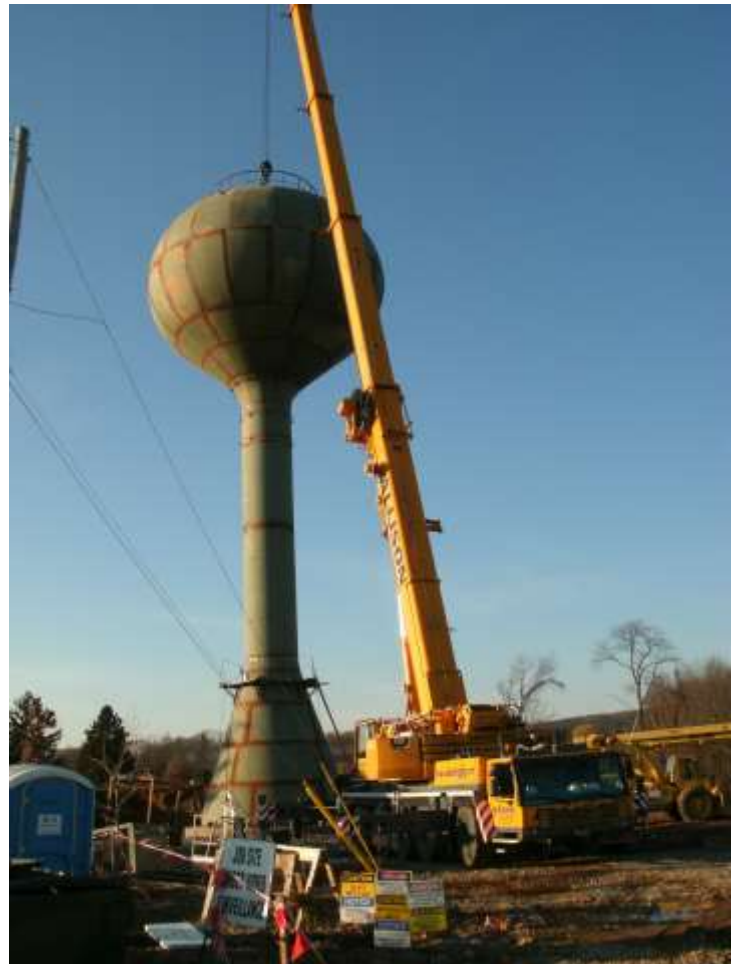
Grey Fox Plaza 200,000 gallon elevated water storage tank installed during summer 2011
