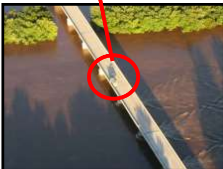
A crew manually tracks river heights using the drop wire gauge during
