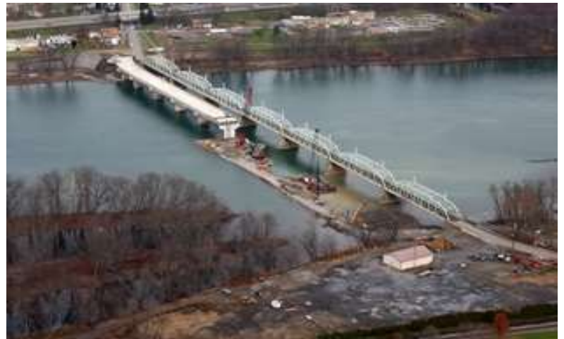
DuBoistown Bridge Replacement
