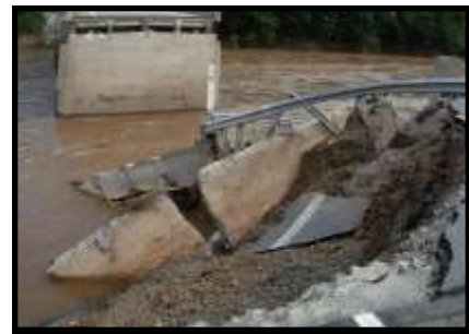
S.R. 973 Bridge, Upper Fairfield Twp.
