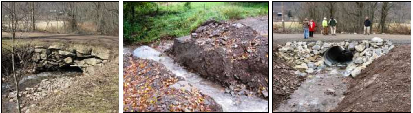
McNett Township Stormwater Improvements: Before Project Initiation, After Flooding Event, and After Project Completion
