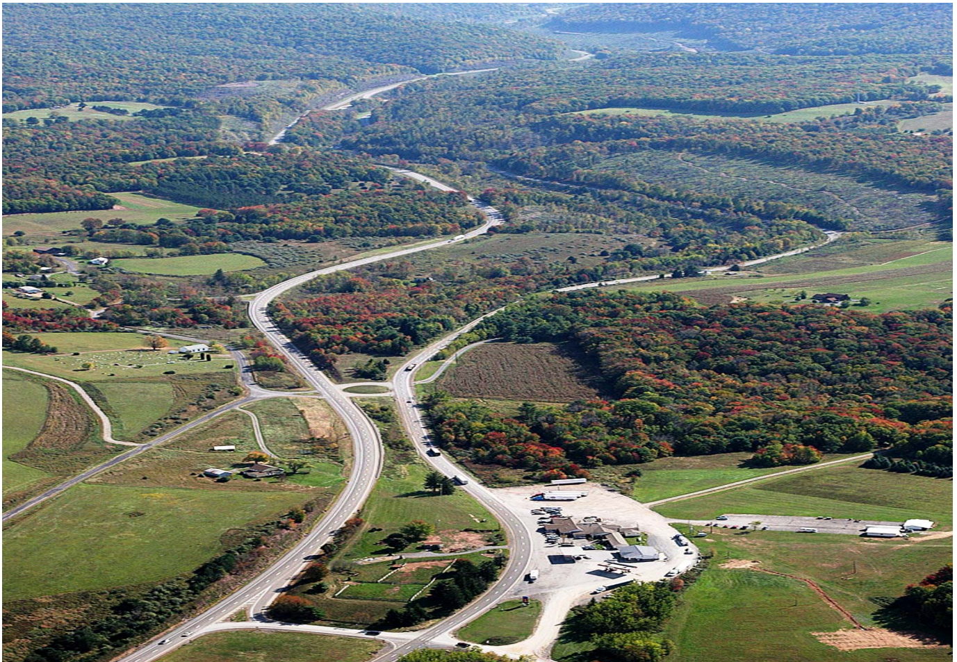
Improved and expanded Route 15 looking south from Fry's Turkey Ranch
