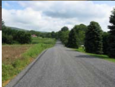
Lehman Road Washington Township Road Reconstruction
