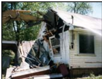
Demolition of flood-damaged home along Lycoming Creek
