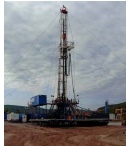
Drill rig at Penn Township site
