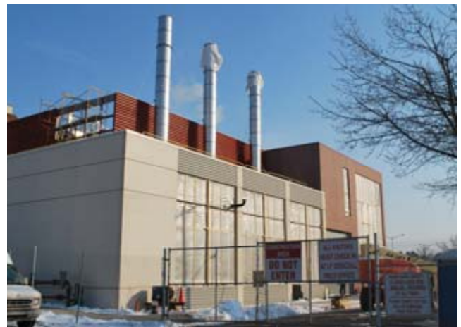
New Energy Service Center
