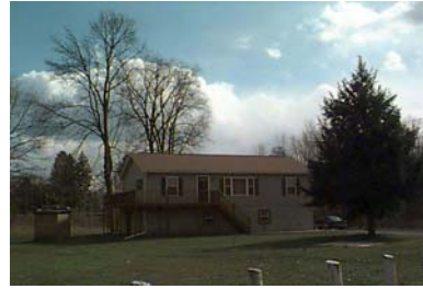
Street Address: 1999 W. Cottage Ave. Parcel ID: 43-011-406 Lat/Long bldg dot: 41 17 8.59 N, -77 3 30.52 W FMV: $123,610
