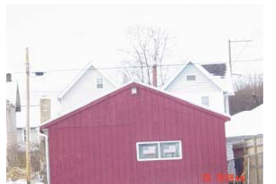
Street Address: 127 Calvert St. Parcel ID: 20-002-516 Lat/Long bldg dot: 41 12 16.86 N, -77 15 38.24 W FMV: $11,460
