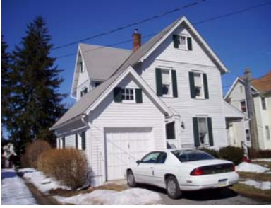
Street Address: 33 Green St. Parcel ID: 39-002-621 Lat/Long bldg dot: 41 12 28.28 N, -76 46 55.86 W FMV: $67,320 1 st floor elevation (ft): 492.7 Lowest grade elevation (ft): 497.7
