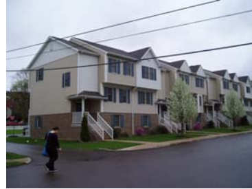
Street Address: S. Market St. Parcel ID: 38-002-216 Lat/Long bldg dot: 41 12 17.82 N, -76 47 15.26 W FMV: 576,000
