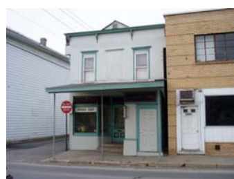
Street Address: 13 W. Water St. Parcel ID: 39-001-222 Lat/Long bldg dot: 41 12 20.34 N, -76 47 13.14 W FMV: $44,130
