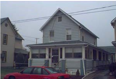
Street Address: 205 Calvert St. Parcel ID: 20-002-408 Lat/Long bldg dot: 41 12 18.19 N, -77 15 36.83 W FMV: $61,770
