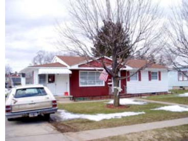
Street Address: 111 Carpenter St. Parcel ID: 38-002-805 Lat/Long bldg dot: 41 12 18.91 N, -76 46 56.39 W FMV: $97,030 1 st floor elevation (ft): 493.9 Lowest grade elevation (ft): 499.1
