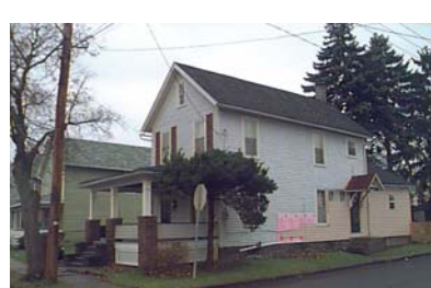
Street Address: 129 Calvert St. Parcel ID: 20-002-517 Lat/Long bldg dot: 41 12 16.93 N, -77 15 37.21 W FMV: $57,160
