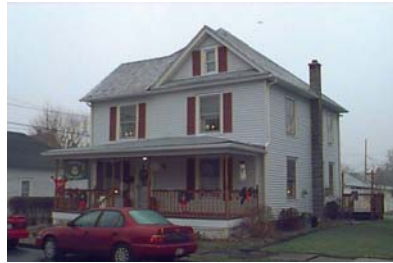
Street Address: 218 Calvert St. Parcel ID: 20-002-419 Lat/Long bldg dot: 41 12 19.57 N, -77 15 35.07 W FMV: $79,950
