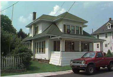
Street Address: 321 Campbell St. Parcel ID: 20-001-418 Lat/Long bldg dot: 41 12 22.35 N, -77 15 22.56 W FMV: $65,060
