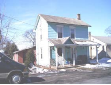
Street Address: 46 Heberling Rd. Parcel ID: 40-004-410 Lat/Long bldg dot: 41 11 49.64 N, -76 47 45.84 W FMV: $80,440
