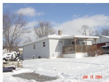
Street Address: 210 Marion St. Parcel ID: 49-005-706 Lat/Long bldg dot: 41 12 31.31 N, -77 15 18.66 W FMV: $60,210
