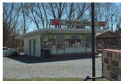
Street Address: 190 Tomb Ave. Parcel ID: 20-001-550 Lat/Long bldg dot: 41 12 14.98 N, -77 15 27.68 W FMV: $76,000
