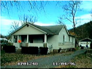
Street Address: 1808 E. Frey Ave. Parcel ID: 43-009-412 Lat/Long bldg dot: 41 15 48.13 N, -77 2 29.80 W FMV: $67,880 1 st floor elevation (ft): 533.9 Lowest grade elevation (ft): 538.6
