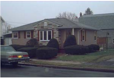
Street Address: 206 Calvert St. Parcel ID: 20-002-422 Lat/Long bldg dot: 41 12 17.97 N, -77 15 35.41 W FMV: $72,530
