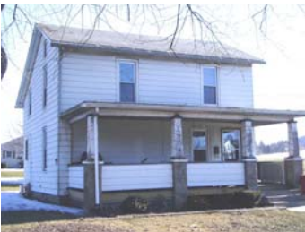
Street Address: 13 Heberling Rd. Parcel ID: 40-004-413 Lat/Long bldg dot: 41 11 51.51 N, -76 47 44.86 W FMV: $51,140
