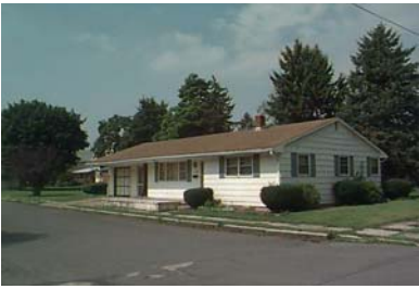
Street Address: 225 Tomb Ave. Parcel ID: 20-001-800 Lat/Long bldg dot: 41 12 19.72 N, -77 15 27.96 W FMV: $69,570
