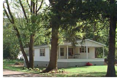
Street Address: 1804 Sweeley Ave. Parcel ID: 43-009-521 Lat/Long bldg dot: 41 15 43.66 N, -77 2 29.10 W FMV: $72,550 1 st floor elevation (ft): Lowest grade elevation (ft): 537.4
