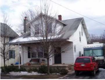
Street Address: 156 E. Water St. Parcel ID: 38-002-824 Lat/Long bldg dot: 41 12 26.32 N, -76 47 46.34 W FMV: $74,890 1 st floor elevation (ft): 493.7 Lowest grade elevation (ft): 497.5
