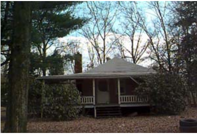
Street Address: 1919 W. Cottage Ave. Parcel ID: 43-011-403 Lat/Long bldg dot: 41 17 15.01 N, -77 3 23.16 W FMV: $29,040
