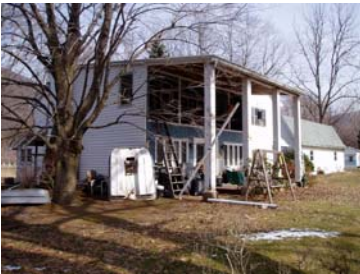
Street Address: 174 Twin Oak Lane Parcel ID: 24-249-150 Lat/Long bldg dot: 41 23 21.09 N, -77 2 47.12 W FMV: $100,970
