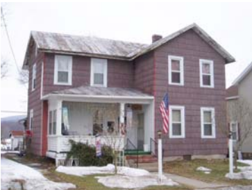
Street Address: 24 N. Market St. Parcel ID: 39-001-128 Lat/Long bldg dot: 41 12 25.93 N, -76 47 17.28 W FMV: $66,680 1 st floor elevation (ft): 487.4 Lowest grade elevation (ft): 491.6
