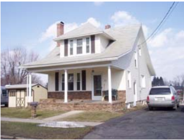
Street Address: 327 W. Penn St. Parcel ID: 38-001-103 Lat/Long bldg dot: 41 12 6.26 N, -76 47 45.88 W FMV: $78,360
