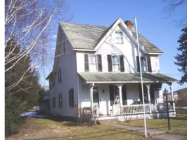
Street Address: 45 Heberling Rd. Parcel ID: 40-393-177 Lat/Long bldg dot: 41 11 49.90 N, -76 47 44.25 W FMV: $139,720
