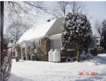
Street Address: 203 Marion St. Parcel ID: 49-005-602 Lat/Long bldg dot: 41 12 29.76 N, -77 15 17.26 W FMV: $50,470
