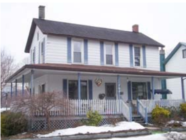
Street Address: 102 N. Market St. Parcel ID: 39-001-130 Lat/Long bldg dot: 41 12 27.21 N, -76 47 17.29 W FMV: $73,780 1 st floor elevation (ft): 487.4 Lowest grade elevation (ft): 490.5
