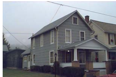
Street Address: 215 Calvert St. Parcel ID: 20-002-411 Lat/Long bldg dot: 41 12 19.50 N, -77 15 36.45 W FMV: $58,290
