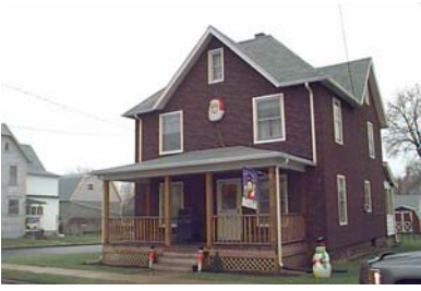
Street Address: 126 Calvert St. Parcel ID: 20-002-518 Lat/Long bldg dot: 41 12 16.61 N, -77 15 35.94 W FMV: $74,350
