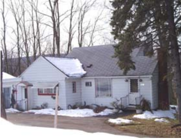
Street Address: 1578 John Brady Dr. Parcel ID: 40-003-219 Lat/Long bldg dot: 41 13 19.31 N, -76 47 45.56 W FMV: $75,480
