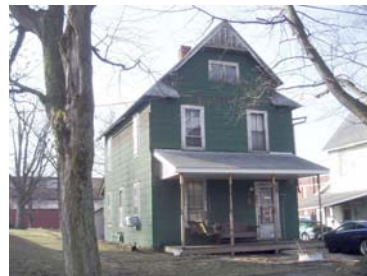
Street Address: 330 W. Penn St. Parcel ID: 37-003-144 Lat/Long bldg dot: 41 12 4.86 N, -76 47 46.68 W FMV: $54,140
