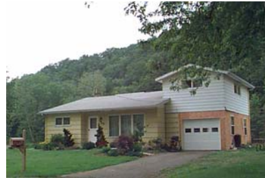
Street Address: 260 Cottage Ave. S. Parcel ID: 43-010-515 Lat/Long bldg dot: 41 15 57.17 N, -77 2 31.45 W FMV: $82,550 1 st floor elevation: 536.2 Lowest grade elevation (ft): 541.8
