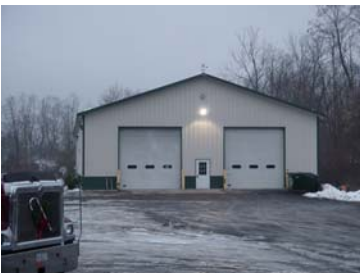
Street Address: Rear Baer St. Parcel ID: 49-005-907.A Lat/Long bldg dot: 41 12 31.18 N, -77 15 12.64 W FMV: $183,080
