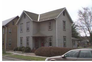
Street Address: 313 Pine St. Parcel ID: 19-002-321 Lat/Long bldg dot: 41 11 53.72 N, -77 15 26.06 W FMV: $68,900
