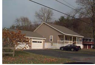
Street Address: 286 Cottage Ave. S. Parcel ID: 43-010-507 Lat/Long bldg dot: 41 16 0.41 N, -77 2 39.56 W FMV: $98,900 1 st floor elevation: 539.9 Lowest grade elevation (ft): 543.8
