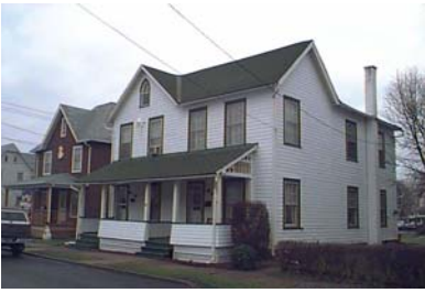
Street Address: 124 Calvert St. Parcel ID: 20-002-519 Lat/Long bldg dot: 41 12 16.19 N, -77 15 36.08 W FMV: $70,830
