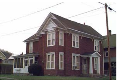
Street Address: 75 Broad St. Parcel ID: 35-005-208 Lat/Long bldg dot: 41 10 14.19 N, -76 52 16.46 W FMV: $67,370
