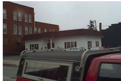
Street Address: 252 Allegheny St. Parcel ID: 20-001-337.A Lat/Long bldg dot: 41 12 10.88 N, -77 15 19.86 W FMV: $23,950
