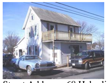
Street Address: 68 Heberling Rd. Parcel ID: 40-004-409 Lat/Long bldg dot: 41 11 48.46 N, -76 47 45.20 W FMV: $65,450
