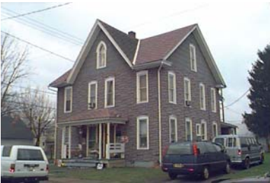
Street Address: 113 Calvert St. Parcel ID: 20-002-512 Lat/Long bldg dot: 41 12 15.42 N, -77 15 37.70 W FMV: $53,510
