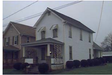
Street Address: 209 Calvert St. Parcel ID: 20-002-410 Lat/Long bldg dot: 41 12 18.76 N, -77 15 36.70 W FMV: $58,410
