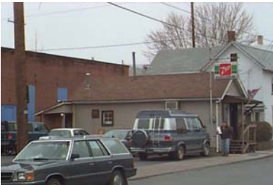
Street Address: 115 S. Broad St. Parcel ID: 20-001-351.A Lat/Long bldg dot: 41 12 8.54 N, -77 15 21.82 W FMV: $13,680
