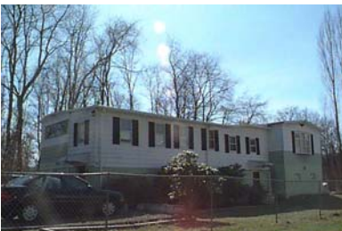
Street Address: 197 Marion St. Parcel ID: 49-005-620 Lat/Long bldg dot: 41 12 27.23 N, -77 15 16.81 W FMV: $32,360
