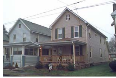
Street Address: 207 Calvert St. Parcel ID: 20-002-409 Lat/Long bldg dot: 41 12 18.50 N, -77 15 36.77 W FMV: $57,320
