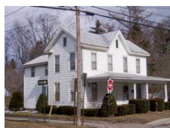
Street Address: 125 E. Penn St. Parcel ID: 38-002-719.A Lat/Long bldg dot: 41 12 9.46 N, -76 46 57.19 W FMV: $88,280
