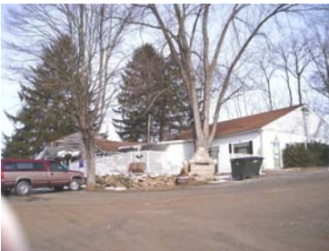
Street Address: 1602 John Brady Dr. Parcel ID: 40-003-218 Lat/Long bldg dot: 41 13 17.99 N, -76 47 43.64 W FMV: $209,670
