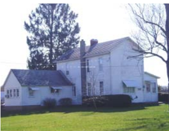
Street Address: 1657 Chippewa Rd. Parcel ID: 40-373-114 Lat/Long bldg dot: 41 12 55.78 N, -76 45 44.96 W FMV: $184,010
