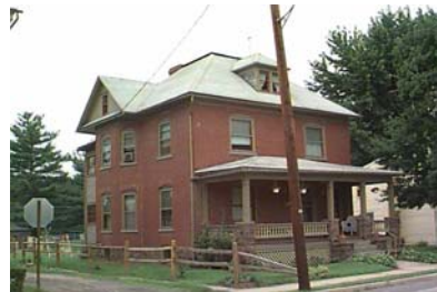
Street Address: 235 N. Main St. Parcel ID: 20-001-123 Lat/Long bldg dot: 41 12 18.13 N, -77 15 11.63 W FMV: $101,580
