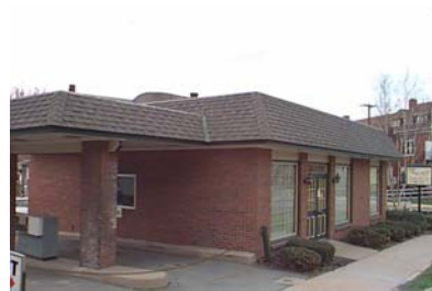
Street Address: 902 Allegheny St. Parcel ID: 21-002-710.A Lat/Long bldg dot: 41 12 15.66 N, -77 15 57.11 W FMV: $81,380
