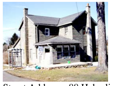
Street Address: 88 Heberling Rd. Parcel ID: 40-004-408 Lat/Long bldg dot: 41 11 47.72 N, -76 47 45.27 W FMV: $71,750
