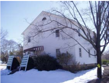
Street Address: 132 E. Mechanic St. Parcel ID: 39-002-601 Lat/Long bldg dot: 41 12 38.46 N, -76 46 54.45 W FMV: $85,240 1 st floor elevation (ft): 489.8 Lowest grade elevation (ft): 493.1
