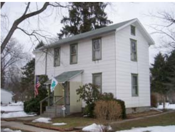
Street Address: 205 N. Market St. Parcel ID: 39-001-314 Lat/Long bldg dot: 41 12 32.20 N, -76 47 16.11 W FMV: $74,790 1 st floor elevation (ft): 484.3 Lowest grade elevation (ft): 488.4
