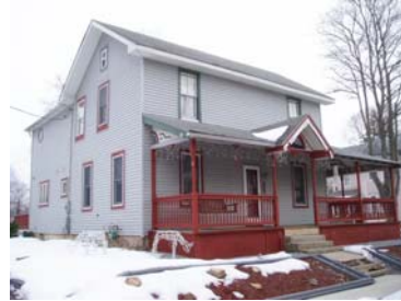
Street Address: 201 N. Market St. Parcel ID: 39-001-315 Lat/Long bldg dot: 41 12 31.31 N, -76 47 16.04 W FMV: $98,140 1 st floor elevation (ft): 486.2 Lowest grade elevation (ft): 491.2
