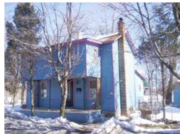
Street Address: 111 N. Washington St. Parcel ID: 39-002-406 Lat/Long bldg dot: 41 12 29.39 N, -76 47 5.28 W FMV: $56,220 1 st floor elevation (ft): 489.3 Lowest grade elevation (ft): 492.2
