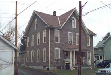
Street Address: 111 Calvert St. Parcel ID: 20-002-511 Lat/Long bldg dot: 41 12 15.20 N, -77 15 37.72 W FMV: $54,240
