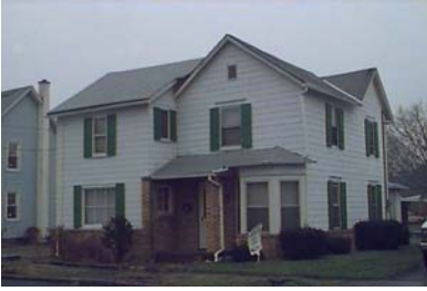
Street Address: 208 Calvert St. Parcel ID: 20-002-421 Lat/Long bldg dot: 41 12 18.51 N, -77 15 35.42 W FMV: $77,160
