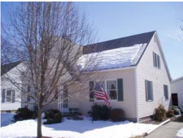
Street Address: 18 Green St. Parcel ID: 39-002-552 Lat/Long bldg dot: 41 12 25.70 N, -76 47 0.66 W FMV: $96,260
