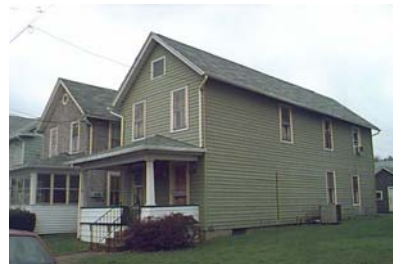
Street Address: 125 Calvert St. Parcel ID: 20-002-515 Lat/Long bldg dot: 41 12 16.52 N, -77 15 37.44 W FMV: $52,020
