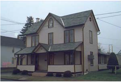
Street Address: 201 Calvert St. Parcel ID: 20-002-407 Lat/Long bldg dot: 41 12 17.65 N, -77 15 37.00 W FMV: $72,080
