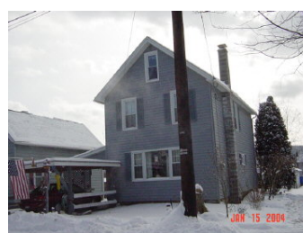
Street Address: 415 Marion St. Parcel ID: 49-005-505 Lat/Long bldg dot: 41 12 32.06 N, -77 15 28.53 W FMV: $69,430
