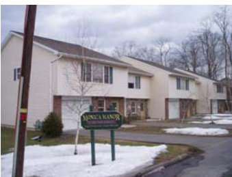
Street Address: 25 Bruner St. Parcel ID: 38-002-611 Lat/Long bldg dot: 41 12 13.77 N, -76 46 59.61 W FMV: $316,800
