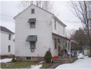
Street Address: 203 N. Main St. Parcel ID: 39-002-206 Lat/Long bldg dot: 41 12 31.83 N, -76 47 9.78 W FMV: $43,130
