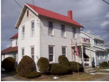
Street Address: 105 Carpenter St. Parcel ID: 38-002-802 Lat/Long bldg dot: 41 12 18.14 N, -76 46 57.70 W FMV: $83,900 1 st floor elevation (ft): 495.4 Lowest grade elevation (ft): 499.0
