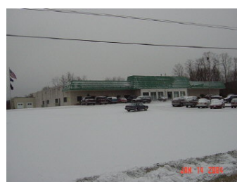
Street Address: 175 A&P Dr. Parcel ID: 49-005-821 Lat/Long bldg dot: 41 12 36.11 N, -77 15 6.48 W FMV: $2,138,240
