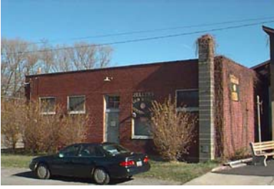
Street Address: 110 Tomb Ave. Parcel ID: 20-001-551 Lat/Long bldg dot: 41 12 12.71 N, -77 15 28.88 W FMV: $21,600
