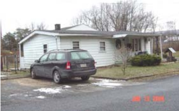
Street Address: Nichols Run Rd. Parcel ID: 49-003-805.A Lat/Long bldg dot: 41 12 15.88 N, -77 16 58.59 W FMV: $76,980
