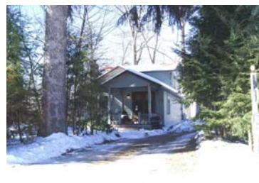
Street Address: 859 Powys Rd. Parcel ID: 15-268-107.A Lat/Long bldg dot: 41 20 47.09 N, -77 5 25.82 W FMV: $53,860
