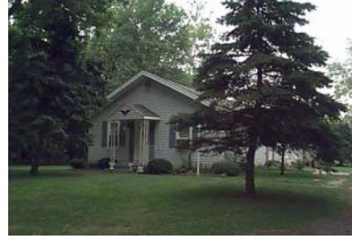
Street Address: 1925 W. Cottage Ave. Parcel ID: 43-011-404 Lat/Long bldg dot: 41 17 14.38 N, -77 3 24.48 W FMV: $62,110
