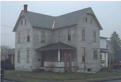
Street Address: 202 Calvert St. Parcel ID: 20-002-423 Lat/Long bldg dot: 41 12 17.53 N, -77 15 35.57 W FMV: $89,900
