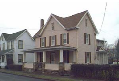
Street Address: 114 Calvert St. Parcel ID: 20-002-520 Lat/Long bldg dot: 41 12 15.72 N, -77 15 36.28 W FMV: $70,430
