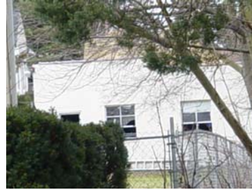
Street Address: 411 Rear Wilson St. Parcel ID: 19-002-302.A Lat/Long bldg dot: 41 11 55.33 N, -77 15 28.44 W FMV: $12,540
