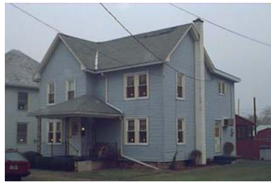
Street Address: 214 Calvert St. Parcel ID: 20-002-420 Lat/Long bldg dot: 41 12 19.08 N, -77 15 35.21 W FMV: $64,710
