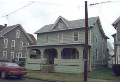
Street Address: 119 Calvert St. Parcel ID: 20-002-513 Lat/Long bldg dot: 41 12 15.84 N, -77 15 37.44 W FMV: $63,520
