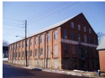
Street Address: 10 S. Market St. Parcel ID: 38-001-301 Lat/Long bldg dot: 41 12 15.76 N, -76 47 17.13 W FMV: $232,360
