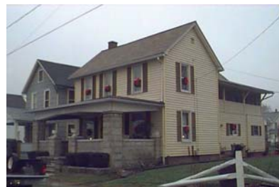
Street Address: 217 Calvert St. Parcel ID: 20-002-412 Lat/Long bldg dot: 41 12 19.75 N, -77 15 36.33 W FMV: $72,910
