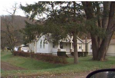
Street Address: 1806 Frey Ave. Parcel ID: 43-009-413 Lat/Long bldg dot: 41 15 47.87 N, -77 2 29.30 W FMV: $63,220 1 st floor elevation (ft): 534.2 Lowest grade elevation (ft): 538.8
