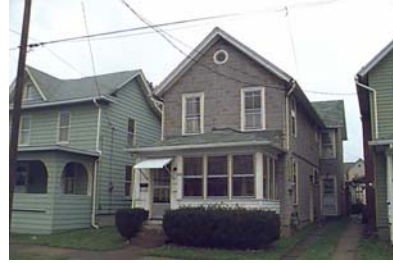
Street Address: 123 Calvert St. Parcel ID: 20-002-514 Lat/Long bldg dot: 41 12 16.20 N, -77 15 37.53 W FMV: $58,010
