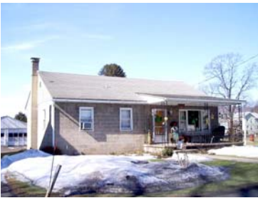
Street Address: 34 Heberling Rd. Parcel ID: 40-004-411 Lat/Long bldg dot: 41 11 50.20 N, -76 47 45.99 W FMV: $65,340
