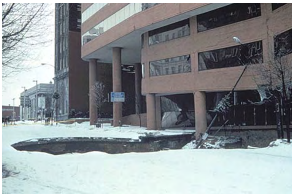
Figure 2: Sinkhole at Corporate Plaza Building in Allentown, Lehigh County, PA, in February 1994 (Photograph by William E. Kochanov - DCNR, 2009)
