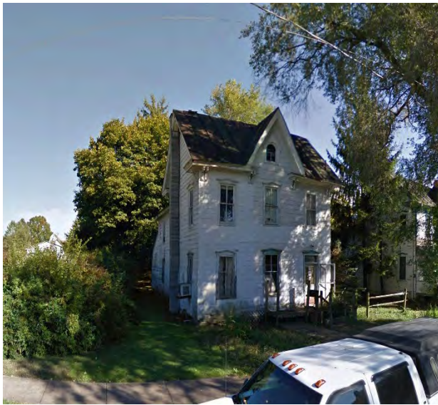
Figure X. No Flood Mitigation Measures In-Place: street view
