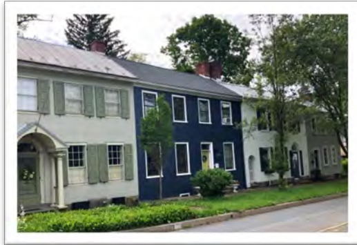
Example Housing within Muncy Borough, 2019
