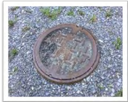
Sanitary sewer cover
