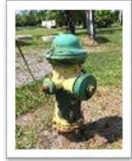
Fire hydrant in the GMA
