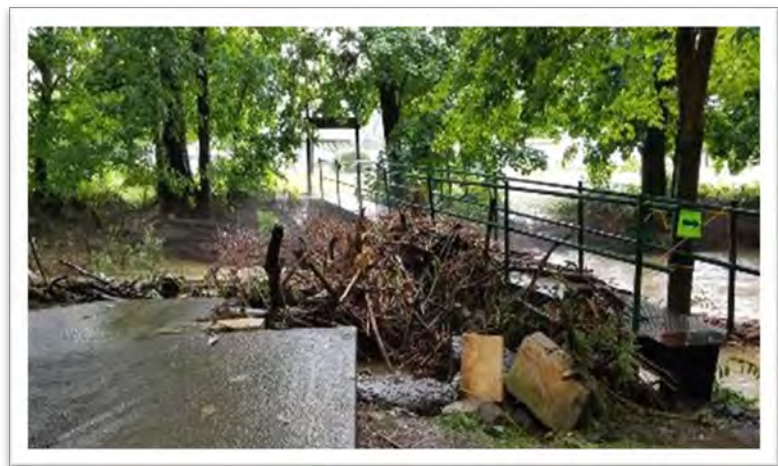
Glade Run Flood Damage in Lions Park, 2018, Source: LDG
