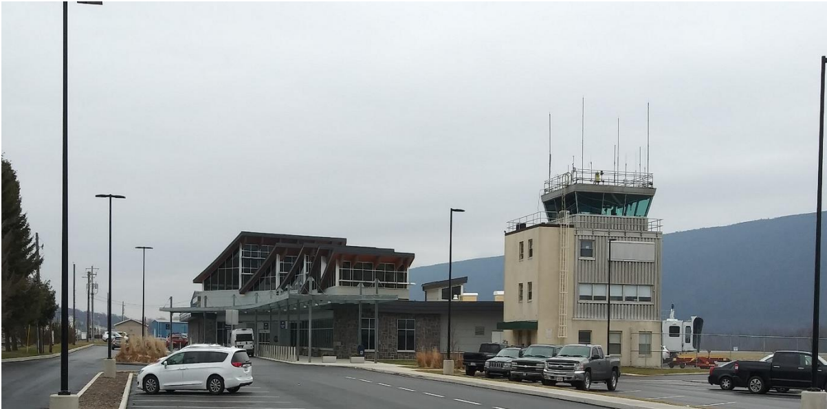
Air Traffic Control Tower, (ATCT)
