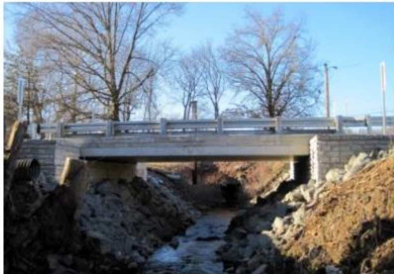
A completed GRS-IBS bridge in Montgomery Park
